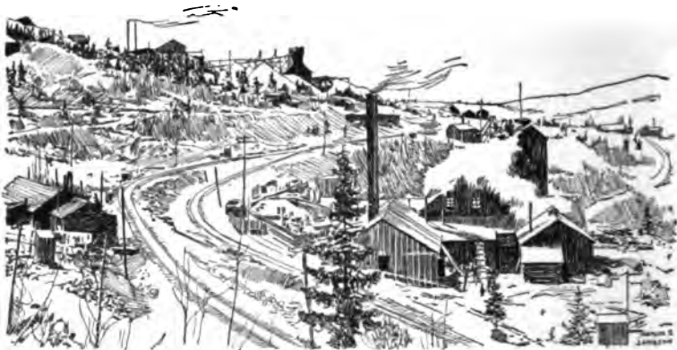
A CRIPPLE CREEK MINE.
